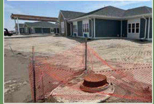
A photo of the new Story Medical Senior Care as it nears completion adjacent to the medical center.
